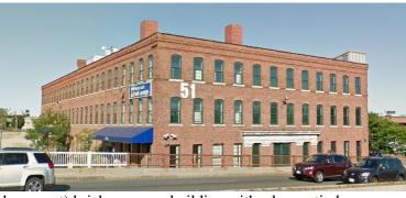
existing structure on the site is a three-story (plus basement) brick masonry building with a heavy timber
